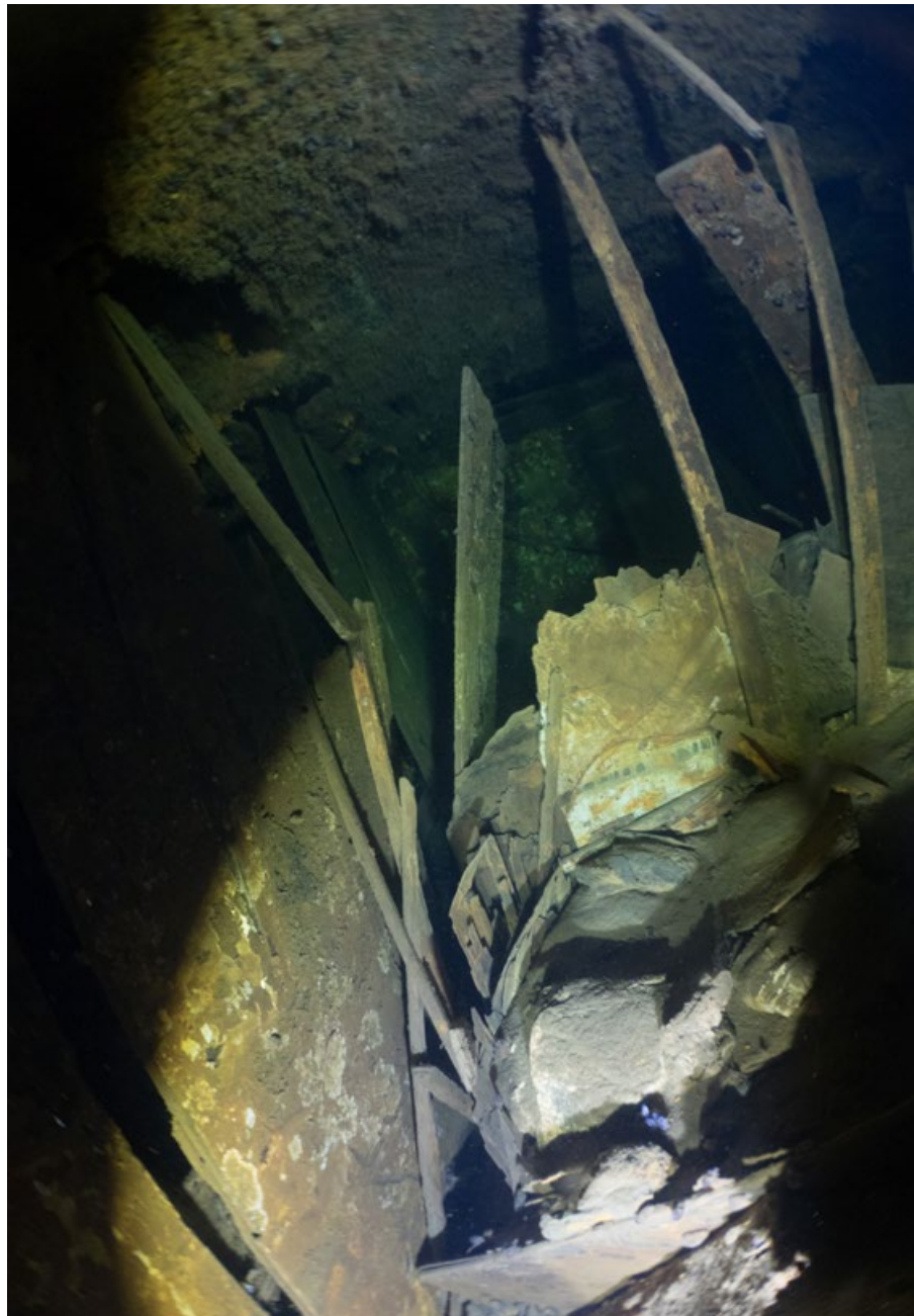
Photo 9. Broken equipment and litter blocking the entrance to the pumping rooms (source: 2018 expedition, © M. Czermański)
